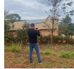
solar power for pump
