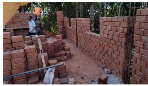
Walls going up
