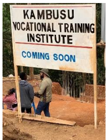
Work in Progress
