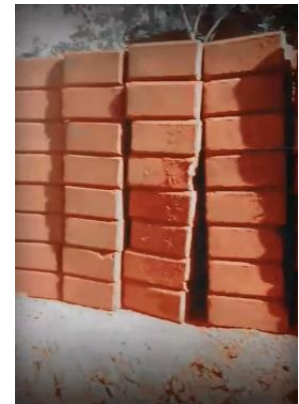
Bricks for above ground construction of Kambusu Vocational Training Institute
