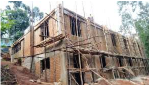
Hillside view: Floors 1 & 2 nearly complete
