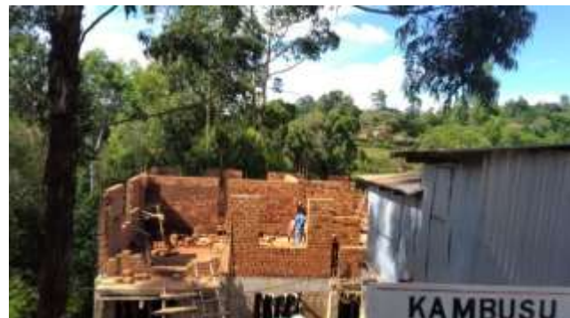
Road view: construction of walls 3 rd floor
